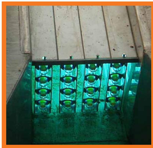
The **SUNLIGHT H-4XE-HO** is a sixteen (16) lamp biologically validated low pressure high output UV disinfection channel system that treats up to 800,000 GPD (for a 200/100 ml) and is designed to treat a 12" water level.
