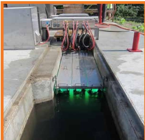
The **GLOW 6000** large flow horizontal amalgam UV disinfection system is designed for large horizontally oriented plants.
